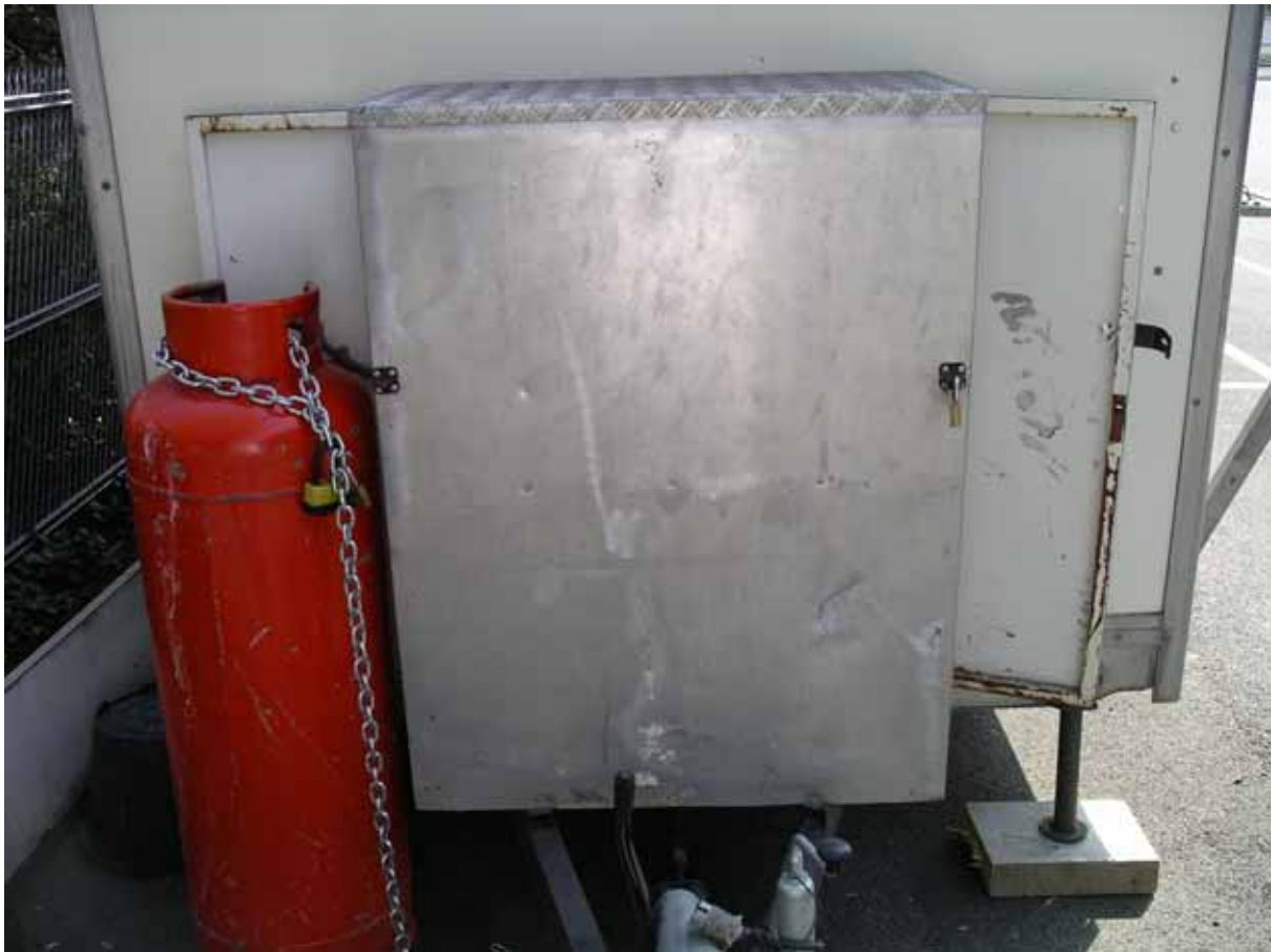
Example of cylinders being secured in the upright position during trading
