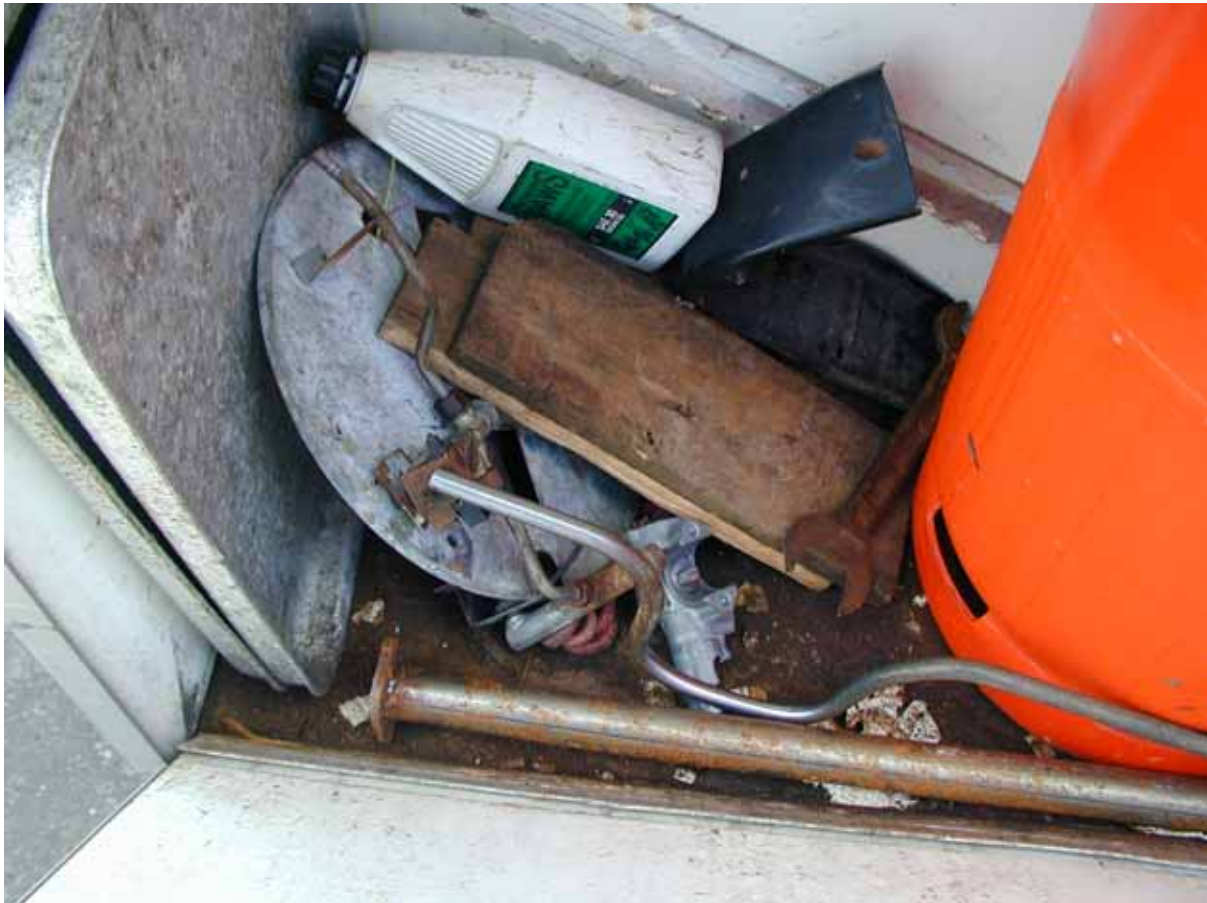
Compartment being used to store equipment other than cylinders, regulators, etc
