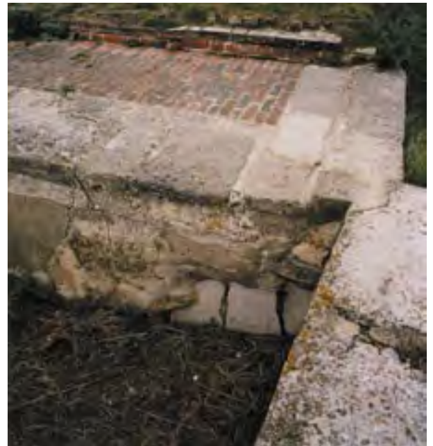
Bembridge limestone blocks on Sidlesham Quay
