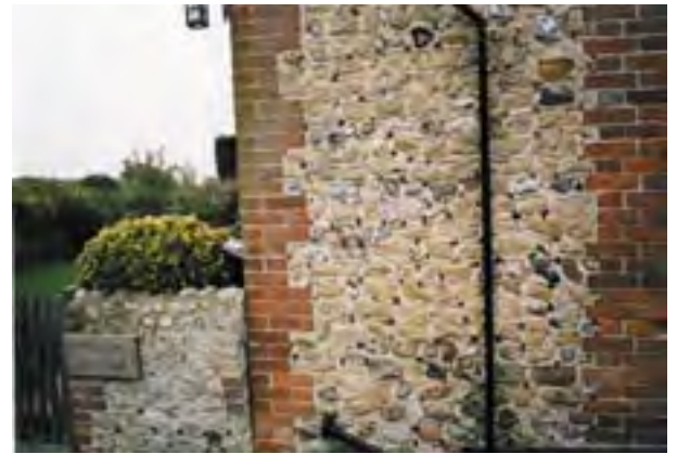
Stone galletting at Johnsons Cottage
