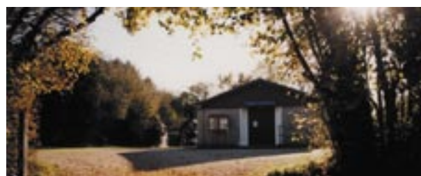
Church hall, Church Farm Lane
