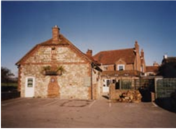
The Anchor Public House
