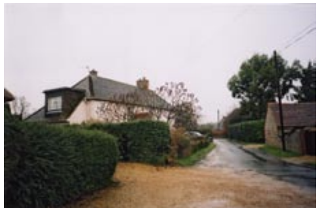
Dormer on side roof slope to Faith's Cottage, Church Lane
