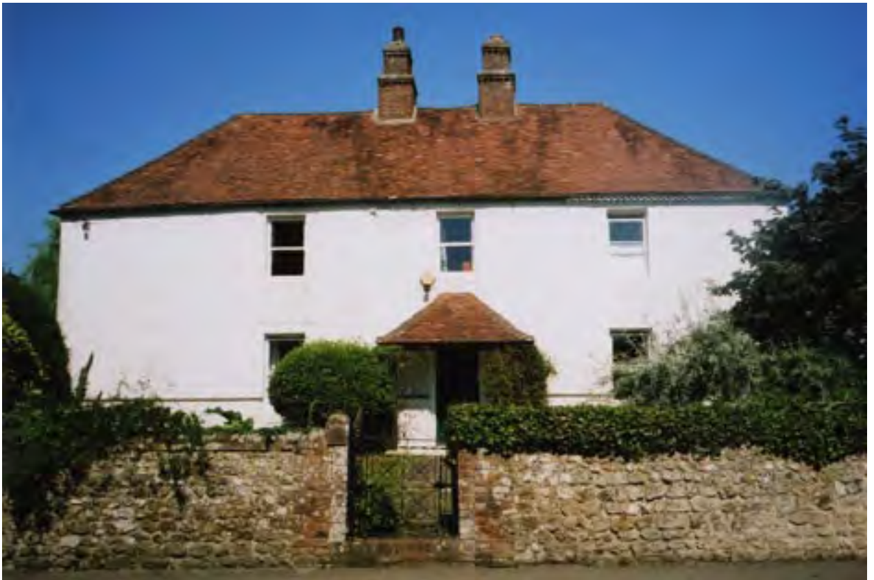
Sandstone wall to Oving Lodge, Church Lane
