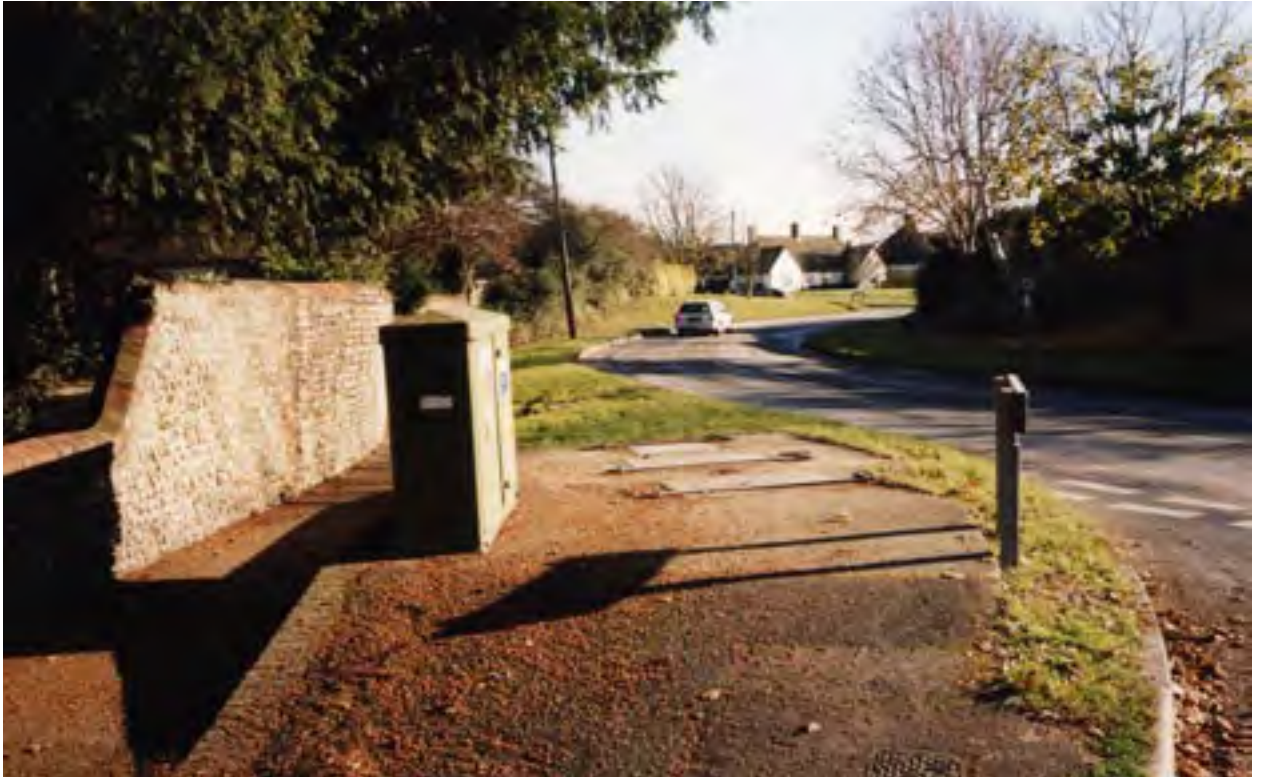
Modern control box in High Street
