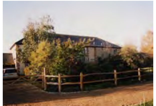
One of the converted barns
