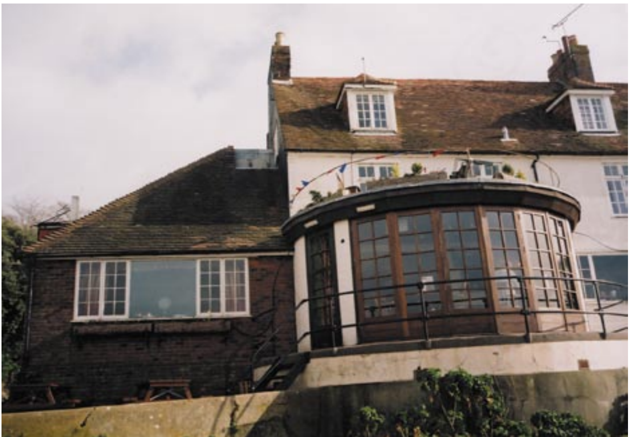
Detail of the rear elevation of the Crown and Anchor Public House
