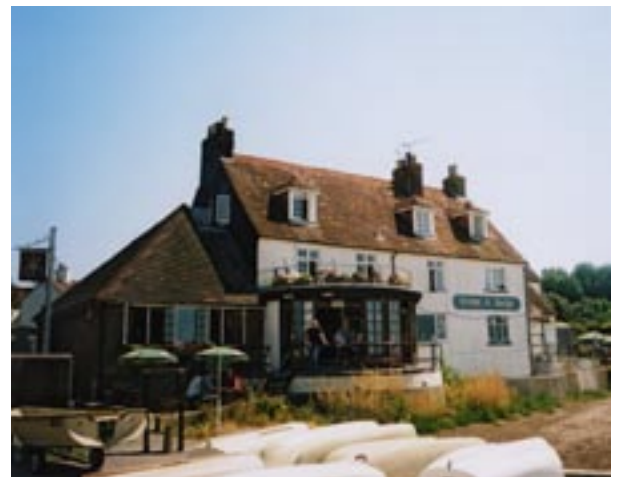
Rear elevation of the Crown and Anchor Public House
