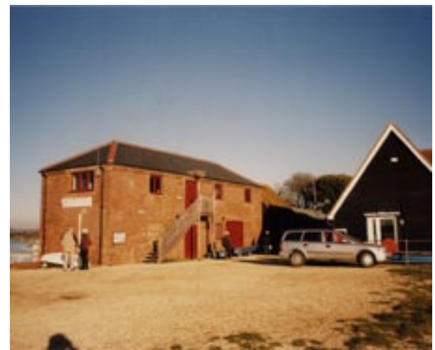
The brick building on Dell Quay makes a positive contribution to the conservation area
