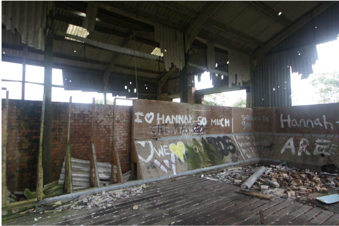
Photo EDP 9: Internal view of derelict farm building in south east corner of field F11
