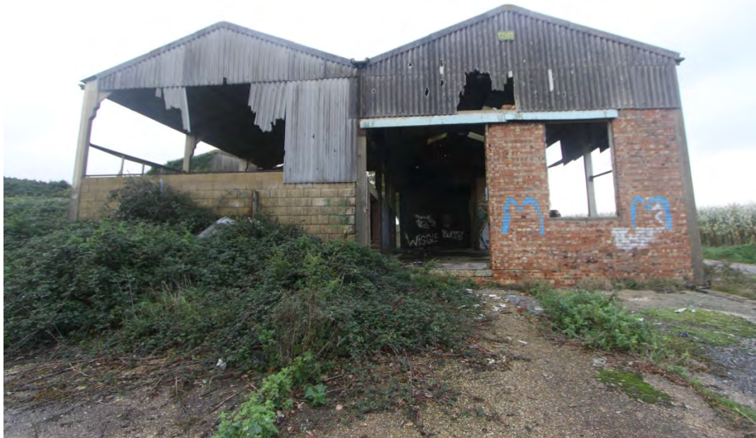
Photo EDP 7: Derelict grain store buildings located in south east corner of field F11
