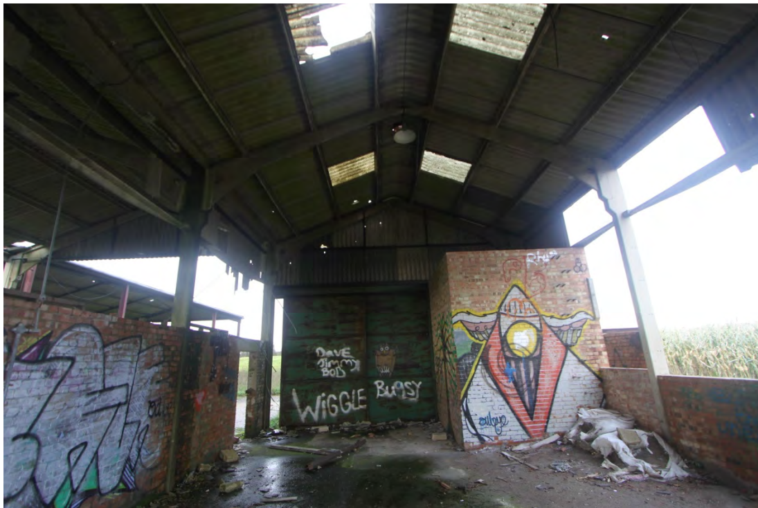
Photo EDP 8: Internal view of derelict farm building in south east corner of field F11
