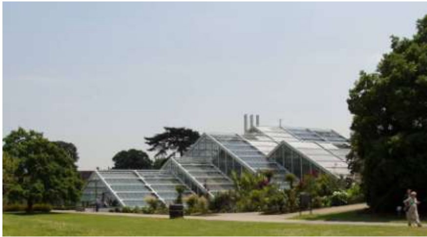
Figure 29 Display Glasshouses - RHS, Wisley
