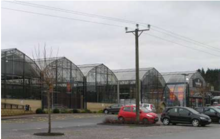
Figure 30 Gothic Roof Profile on Glasshouse Used for Retail Sales
