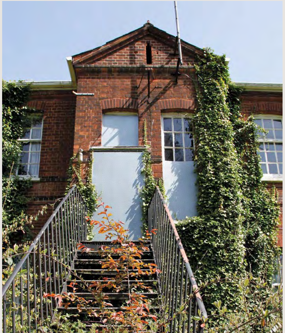
Unmanaged climbers can grow up onto roofs and into gutters, dislodging roof slates and blocking rainwater drainage.
