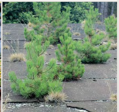
If tree seeds fall on roofs and get established, their roots can exploit cracks in the covering and open up channels for water to get into the building.
