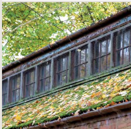
A build-up of dead leaves and moss encourages damp and can block gutters and downpipes.
