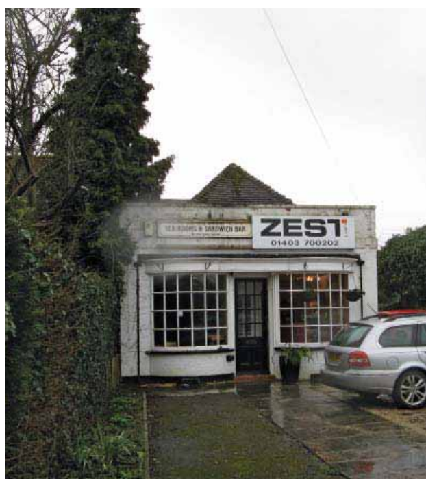
Former tea rooms and ‘Zest’, Petworth Road
