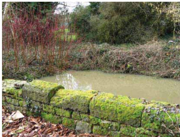
Stone wall to pond at Park Cottage
