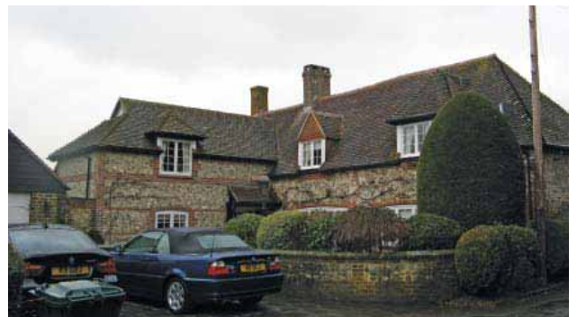
Nos. 70 and 71 Church Lane (now one house)
