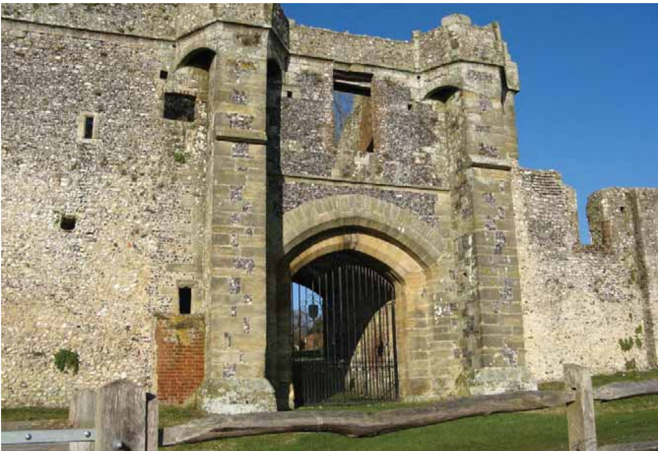
Ruins of Halnaker's 14th century former manor house, in the proposed extension to the adjoining Halnaker Conservation Area
