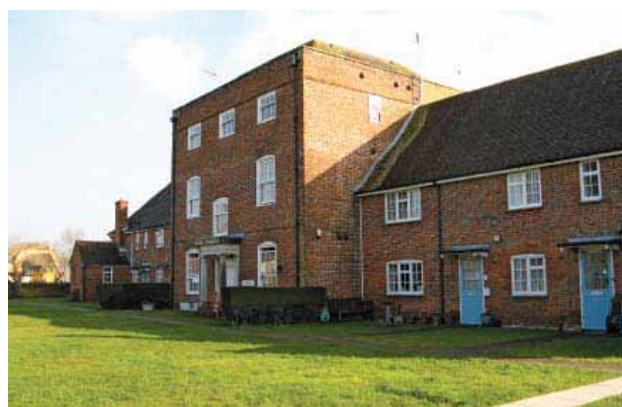
Rear view of the Duchess of Derby's Almshouses, Boxgrove
