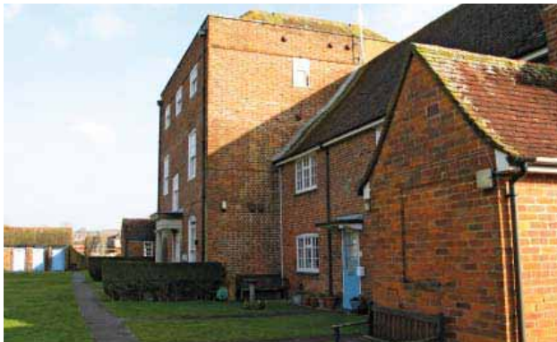
Rear view of the Duchess of Derby's Almshouses
