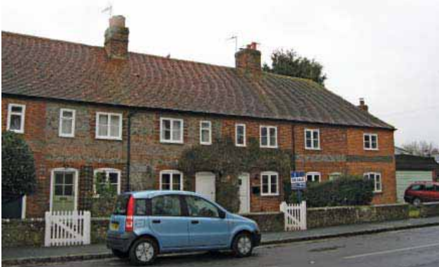
These brick walls need to be protected from demolition (The Street)
