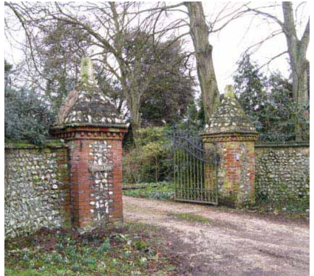
Gate piers to Priory Gate
