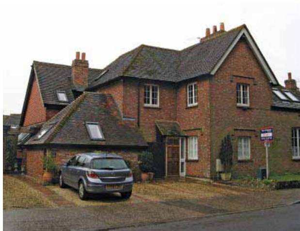
The removal of front boundaries to create car parking areas in The Street
