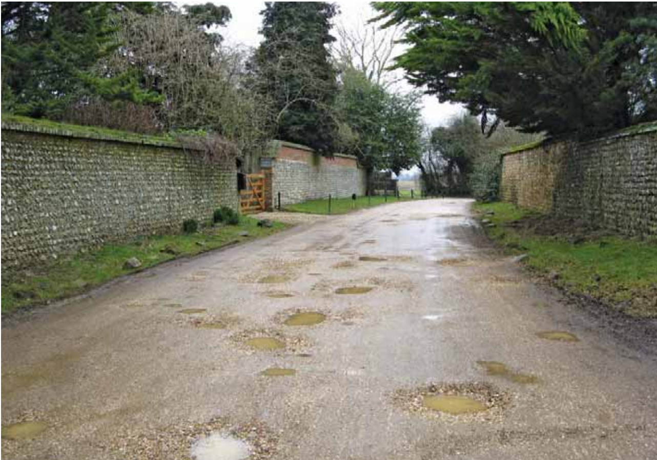
Flint walls line the driveway to the Priory (the road surface has since been repaired)
