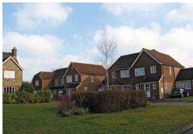
Delete these modern houses in Priors Acre from the conservation area
