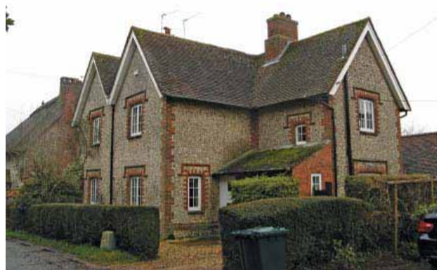
'Duchess' cottages in Church Lane
