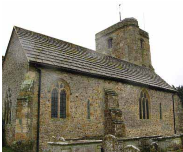
Local stone walling in St John's Church, with a Horsham stone slate roof
