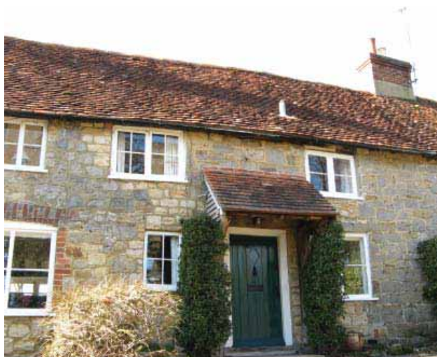
Ivy Cottage is timber-framed but the front elevation is faced in winklestone
