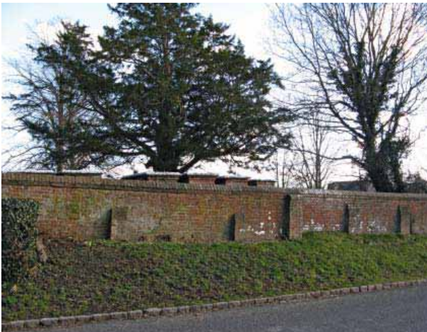
Brick wall to St John's Churchyard
